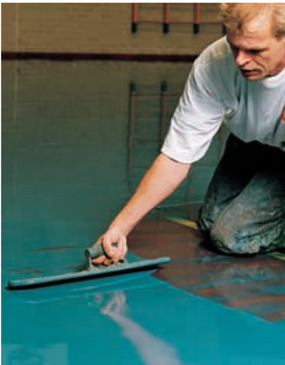
A seamless polyurethane sports floor finish constructed from two 1mm-thick layers over a reinforcing mesh on top of resilient prefabricated granulated rubber sheets that are bonded to the subsurface. The playing surface is given a matt finish and court markings are applied with polyurethane paint.
