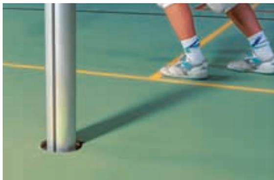
Removable section in polymeric floor for volleyball posts.
