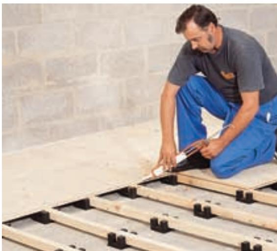
Plywood decking fixed to battens suspended on rubber pads to conform to BS 7044.
